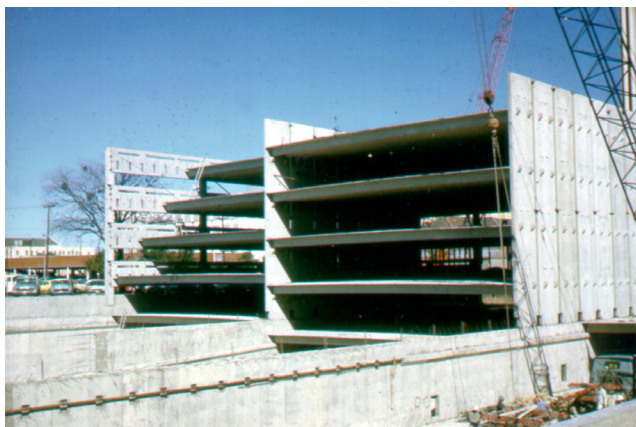
"Stack Walls" Along the Ramp Under Construction
