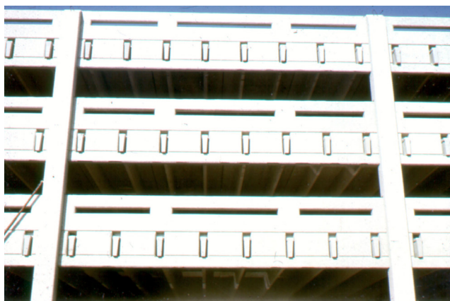
Unique Double Tee Support Used at the Exterior Spandrel Beams
