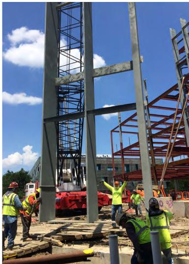
in the plant and ship in 10'-0" wide sections. The sections were composed of the three steel plate columns and all of the horizontal struts and beams welded to the columns in the plant. This would leave only lifting, bracing, and attaching the three column panels in the field.
