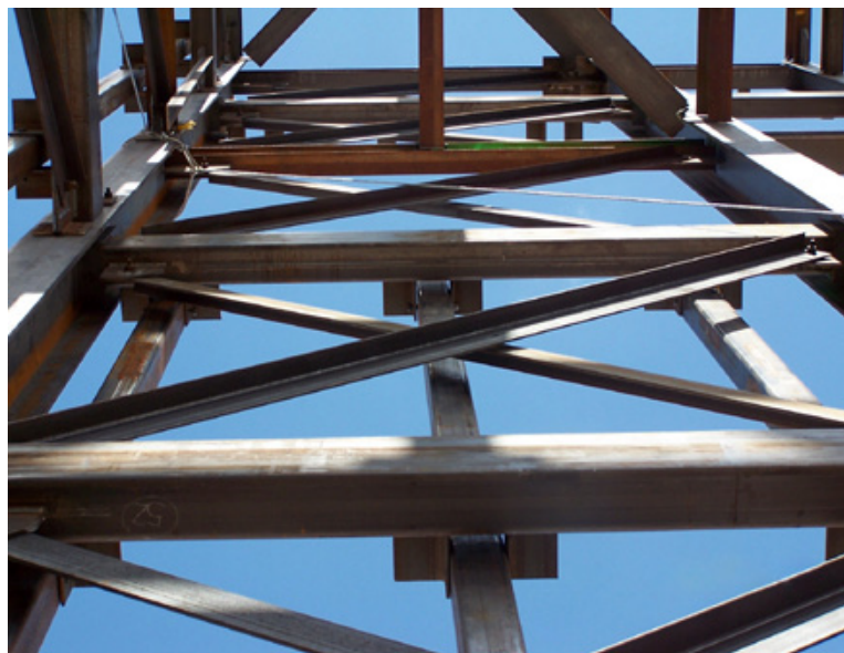
▲ Full-height cross-braces at the corners provide stability to the Urban Lantern tower.
