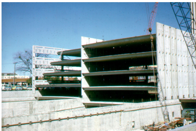
"Stack Walls" Along the Ramp Under Construction
