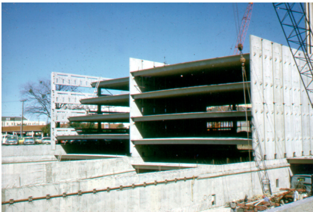
"Stack Walls" Along the Ramp Under Construction
