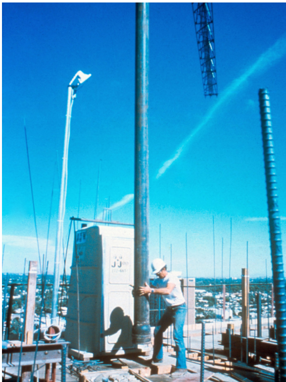
Figure 17 Installation of Vertical Plumbing Riser
