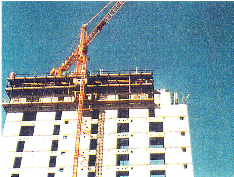
Figure 29 Reduced Form Above Offset in Core
