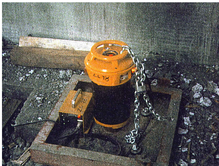
Figure 21 Laser at Ground Level to Guide Slipforming
