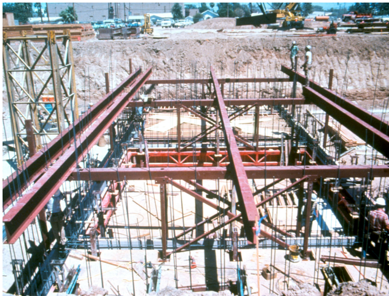
Figure 9 Jacking Grid
