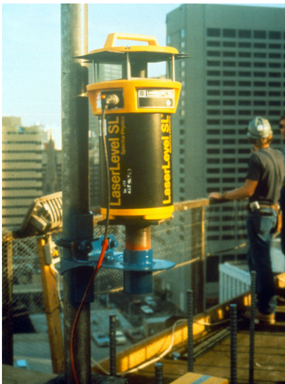
Figure 23 Laser at Corners of Form
