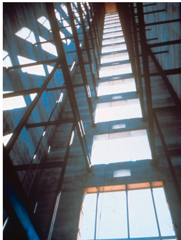
Figure 24 Structural Steel Erected From Slipform
