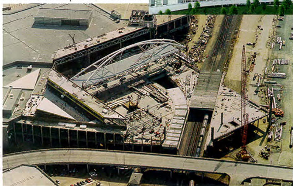
OBSTACLES Convention center expansion spans six rail lines and two city streets.
