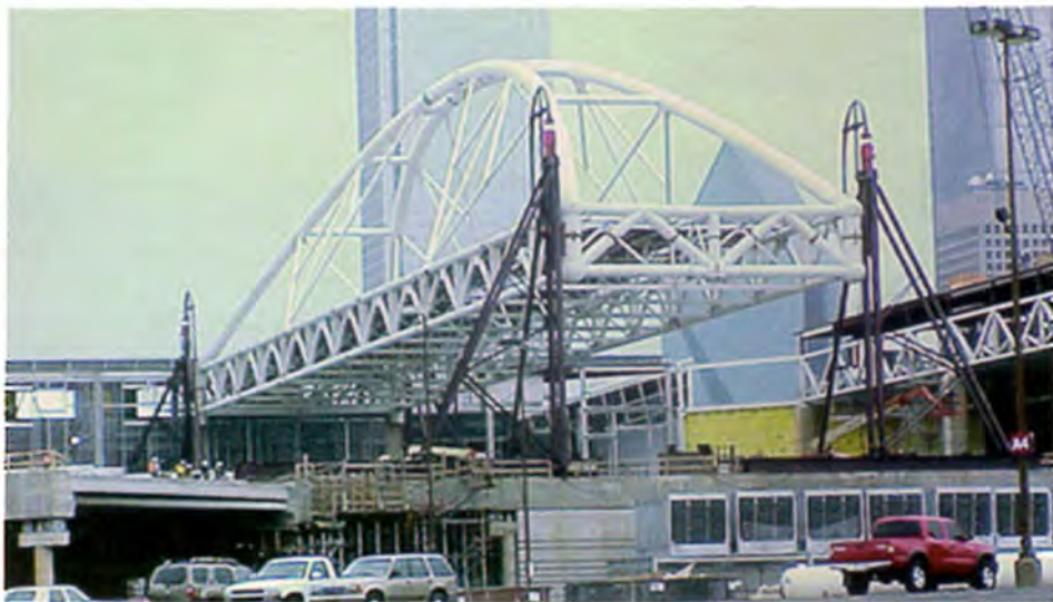
SUSPENDED Bowstring trusses will support a 200,000-sq-ft column-free space.
