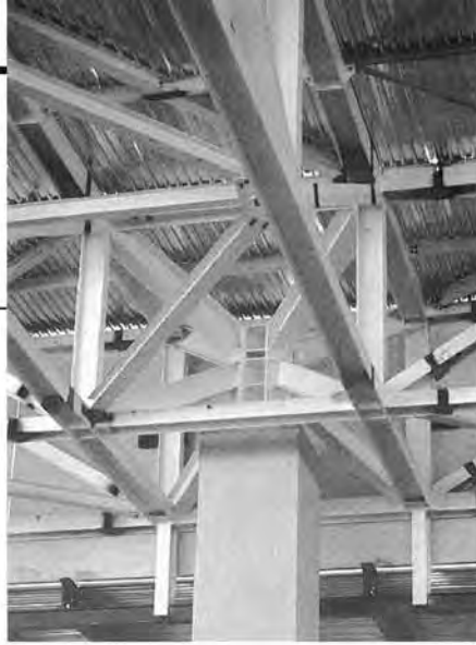
Roof of two-part addition to Dallas Convention Center is supported by steel box beams that meet at "nose cone" connections (right).
