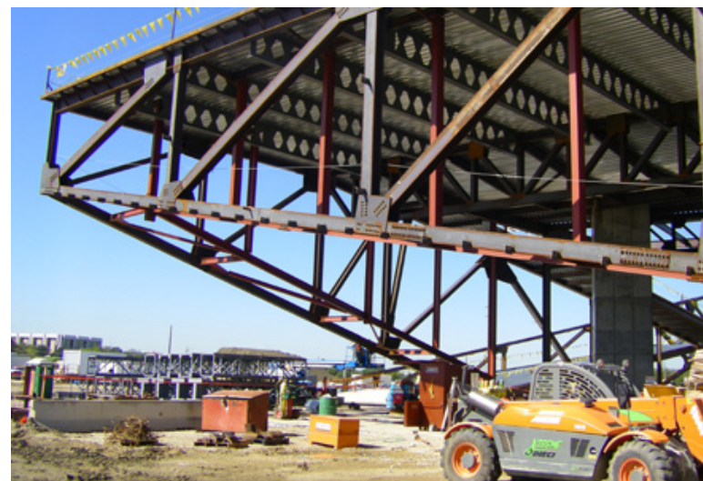
▲ Cantilevering the floor structure over the two main entries allowed the area to remain column-free.
